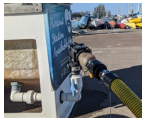
A gravity-drained dump station manually connected to a pumpout unit’s infrastructure by attaching the pumpout unit’s hose to the dump station waste fitting Photo by SFEP
